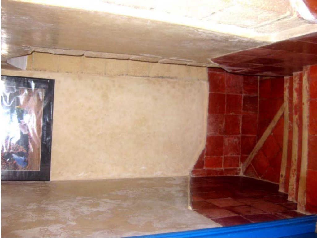
Hotel Riad Tahraouia, 31 Rue Agadir in Essaouira
