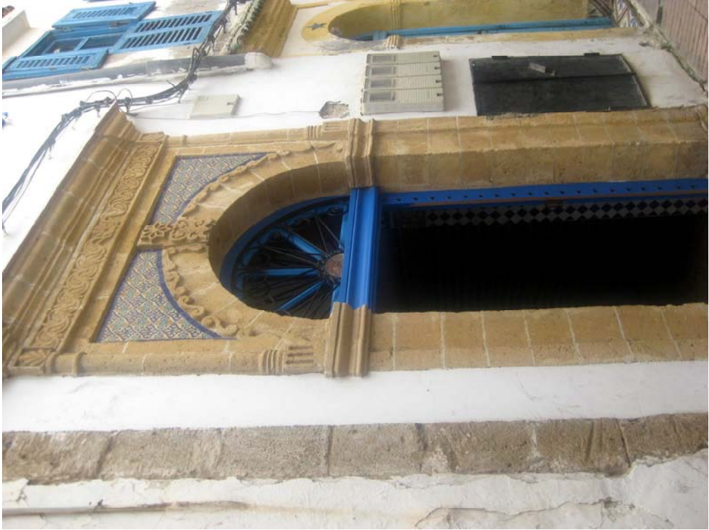
Hotel Riad Tahraouia, 31 Rue Agadir in Essaouira
